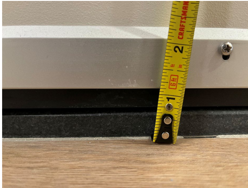
Figure 2: Unit 412's entry door threshold measuring above 1/4 inch without a sufficient bevel
