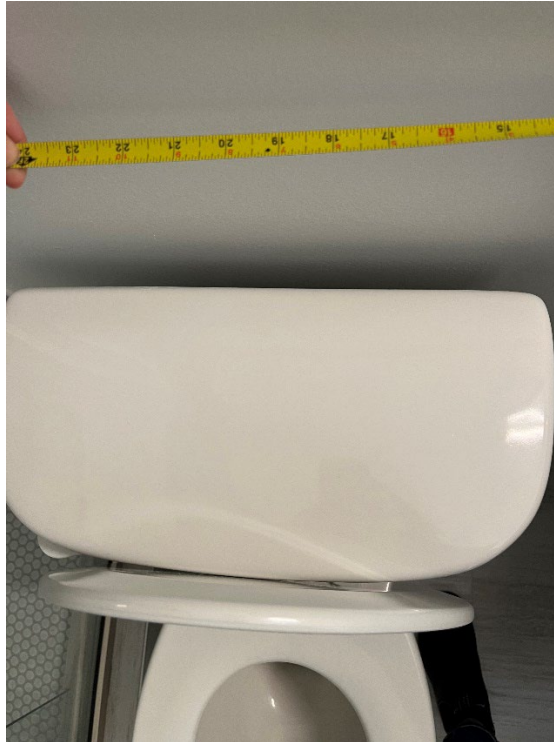
Figure 19: Unit 302 toilet centerline of approximately 19.5 inches.
