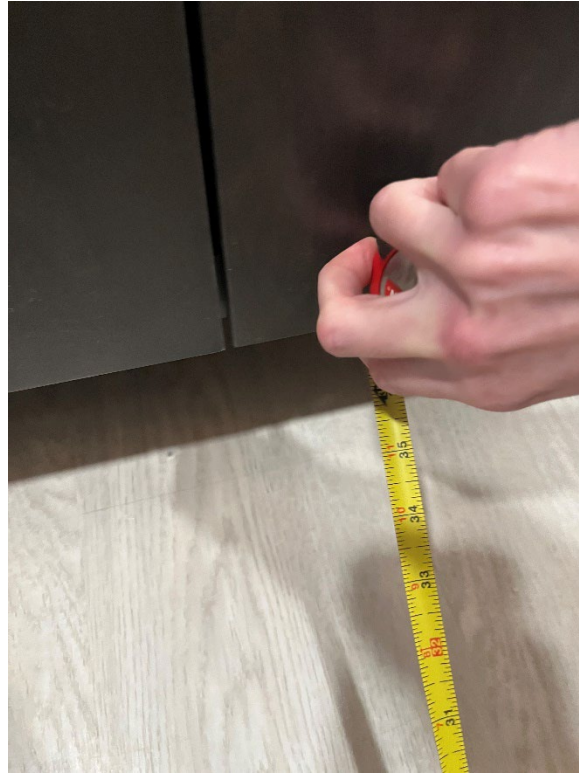
Figure 14: Unit 409 measuring approximately 36 inches of clearance between kitchen counters and appliances.
