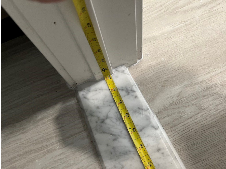
Figure 5: Unit 302 bathroom door measuring approximately 23 inches.
