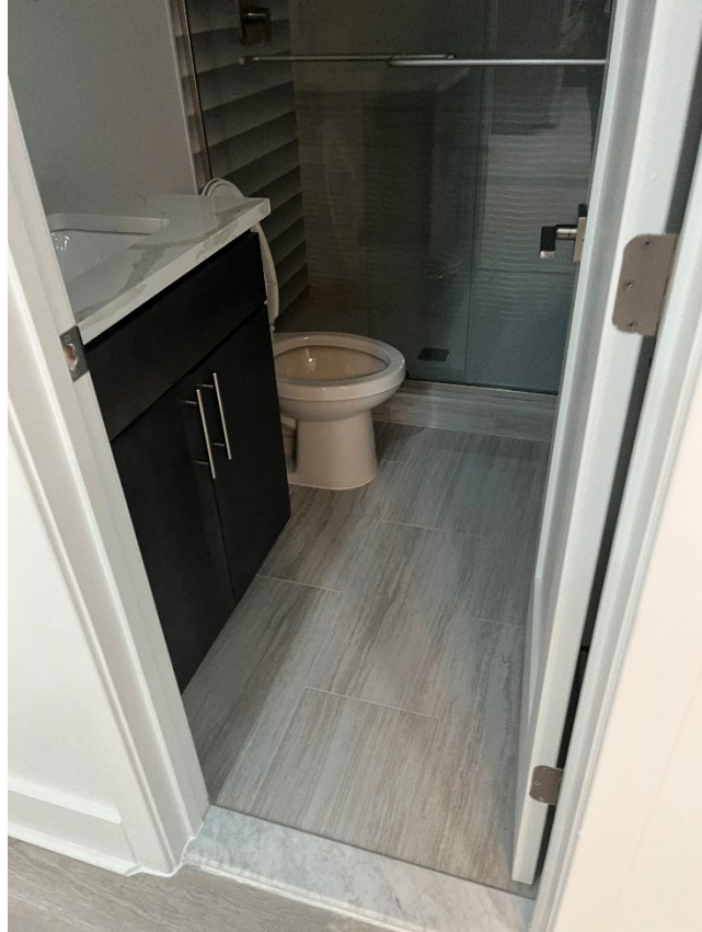
Figure 17: Unit 409 bathroom featuring less than 30" x 48" of clear floor space.
