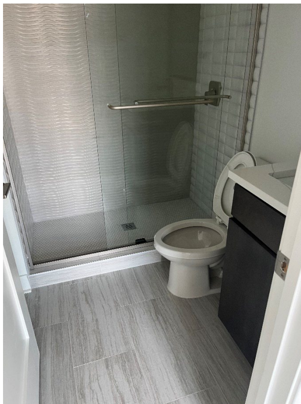
Figure 17: Unit 409 bathroom featuring less than 30" x 48" of clear floor space.
