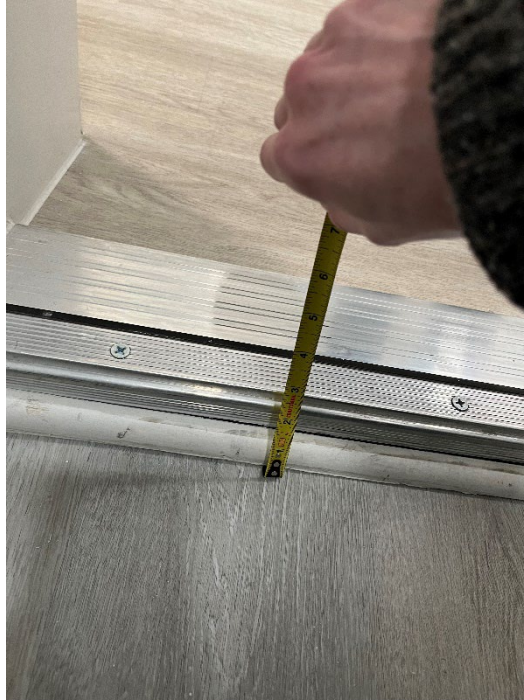
Figure 8: Unit 411 primary exterior door threshold measuring approximately 2 inches.
