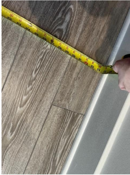
Figure 4: Unit 302's hallway narrowed to 34 inches.
