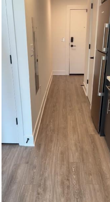
Figure 6: Unit 308's hallway narrowed to 34 inches.
