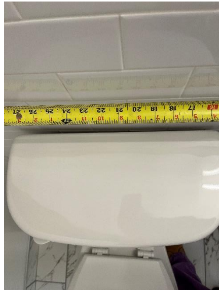
Figure 3: Unit 308 toilet centerline of approximately 21 inches.
