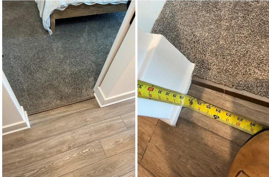
Figure 1: Unit 204 bedroom door measuring approximately 27.5 inches.
